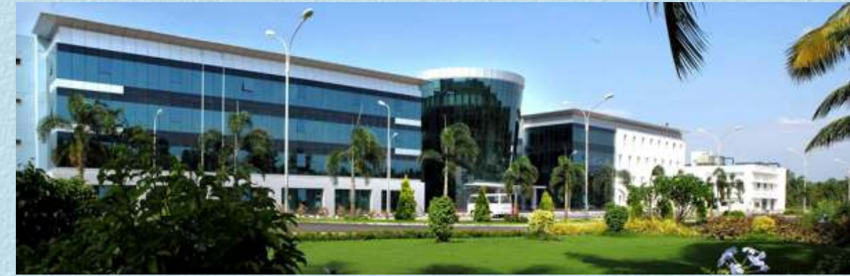
'Chaithanya' 2.4 lakhs sq.ft. SEZ Building
