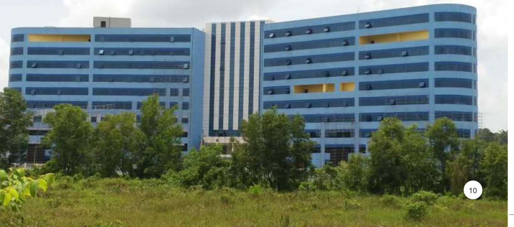
4 lakhs sq.ft. IT building 'Jyothirmaya' nearing completion
